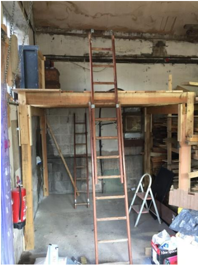
Upper storage deck takes shape
